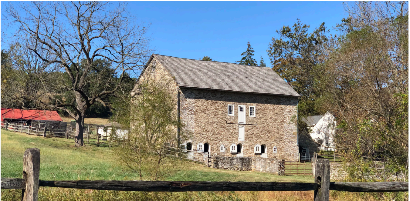
Historic barn along Green Valley Road.
